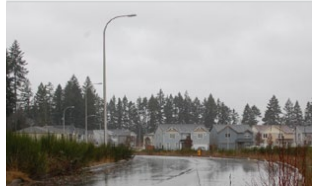
Deschutes River Highlands Phase 2
